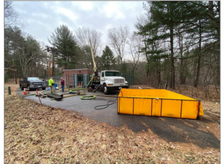
Main Street Well Rehab
